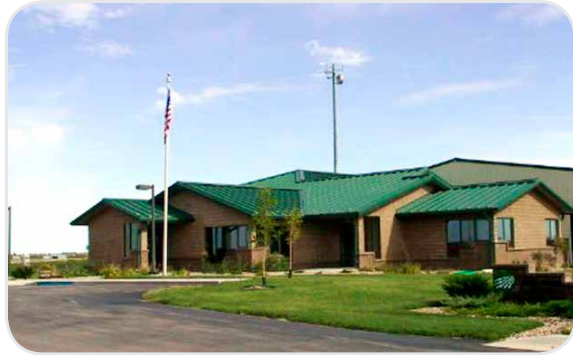
Wall, SD Office
