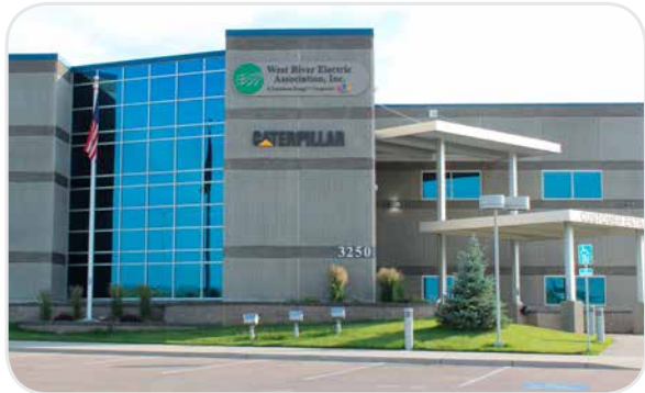
Rapid City Office
